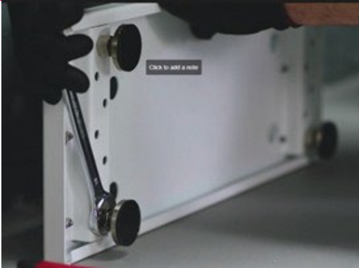
Figure 6: Floor stand—tightening the nut
